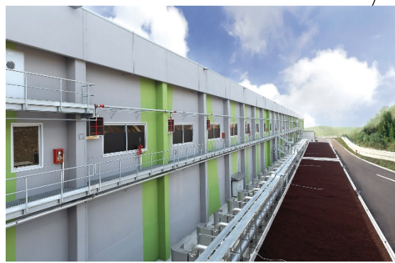
(2) BIOFILTER FOR THE PROCESS AIR CLEANING AND ODORS ABATEMENT
